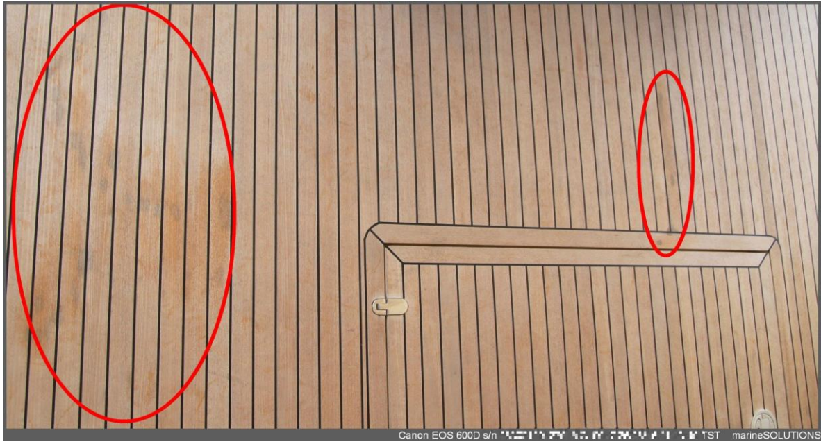
Dark coloured stains on the cockpit teak deck.
