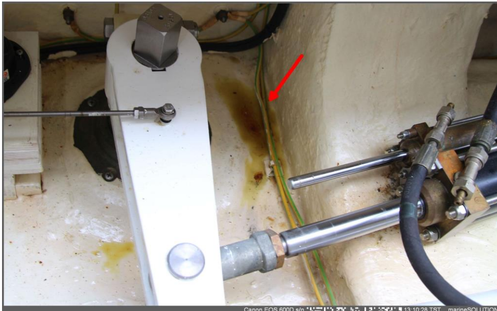
Oil leak traces at the starboard side rudder arm.
