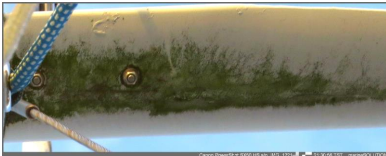
Above: Moss growth on the starboard lower spreader
