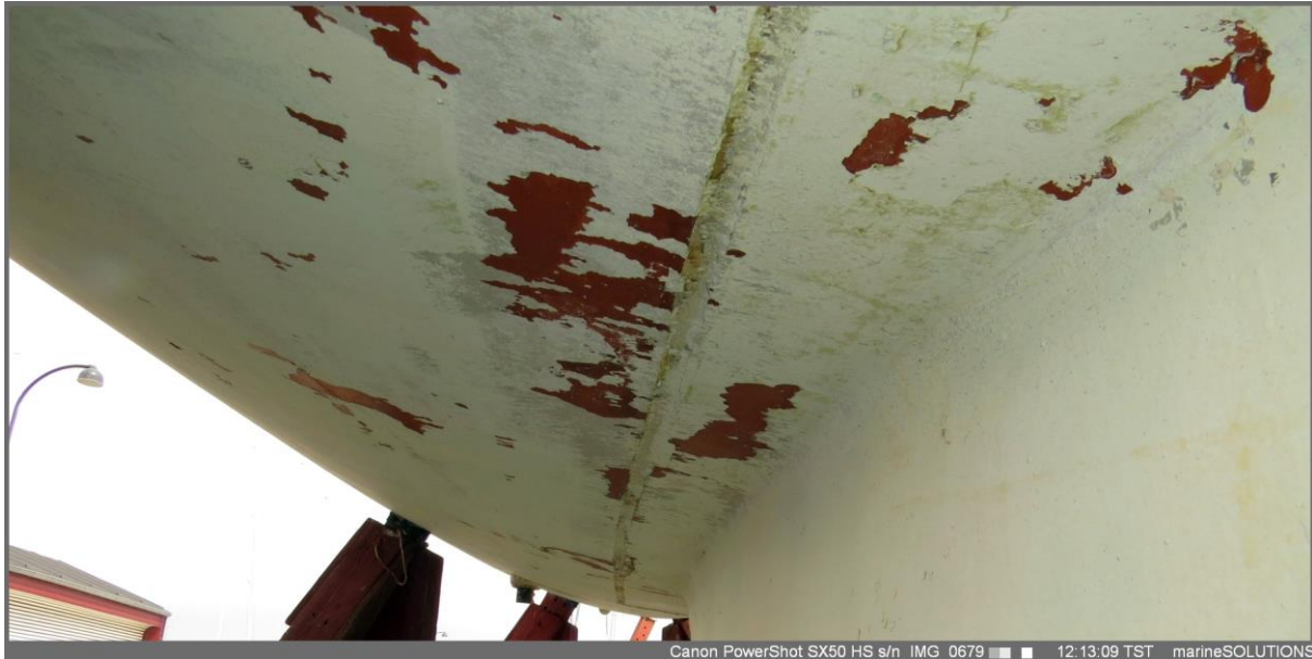
Above: Flaked off (red) areas on the submerged hull and the layer underneath of present antifouling.
